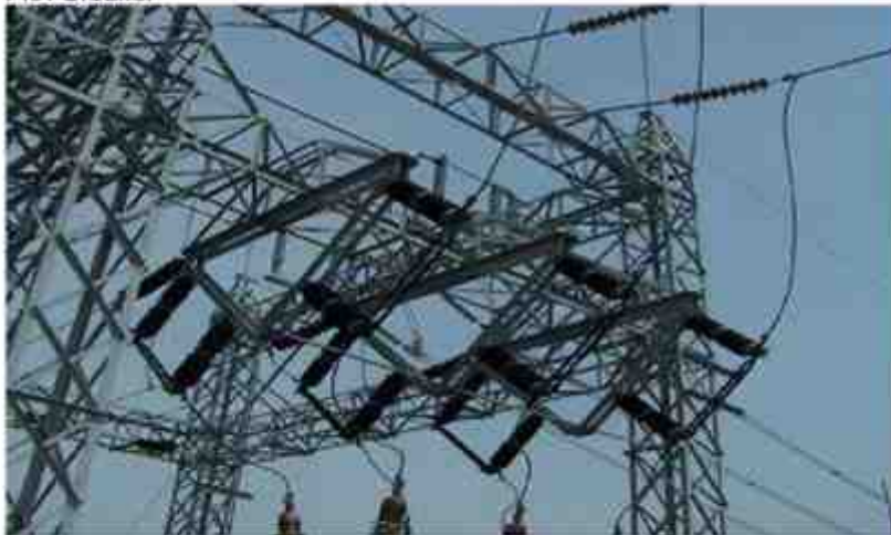
Pic 2 disconnect switches 102 and 106
