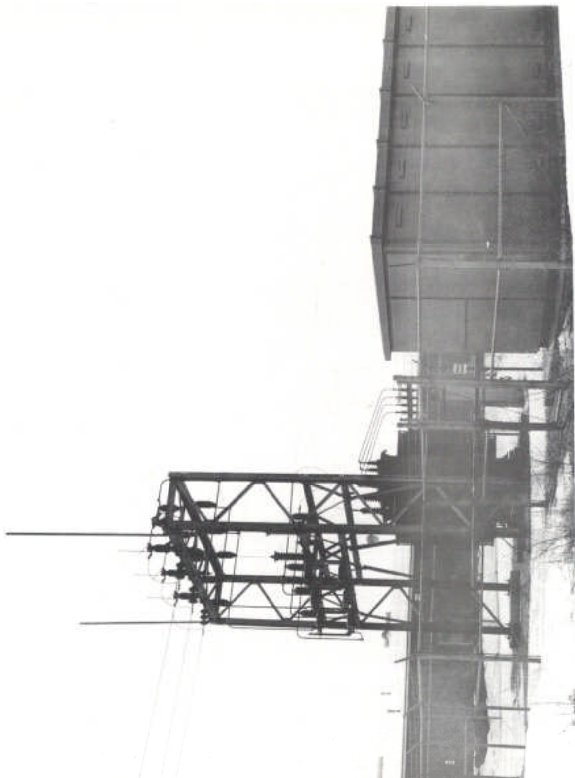
Typical 34.5 KV Station
